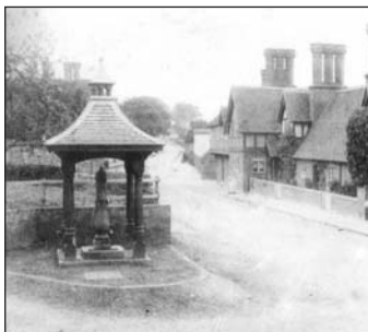
The Pump before the Station Road junction was moved to the north side
